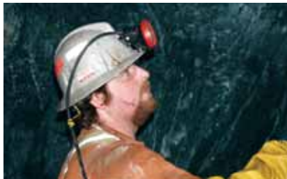
BRAD MULHALL SCALES HINGE MINE STOPE 9780-04 WHILE PREPPING TO BOLT AND SCREEN THE AREA.
