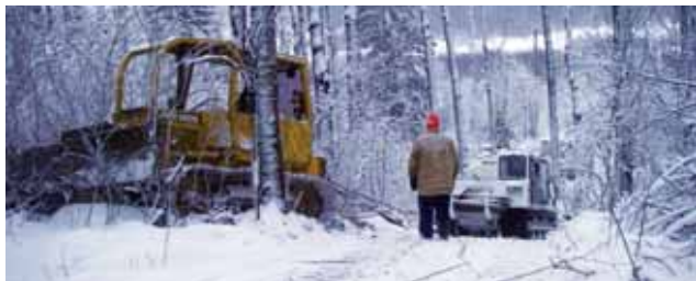
GEOTECHNICAL DRILLING PROGRAM AT MAKWA
