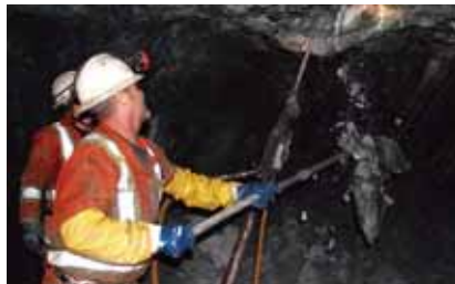
DENNIS CHRAPON SCALES HINGE MINE STOPE 9780-04 WHILE PREPPING TO BOLT AND SCREEN THE AREA.
