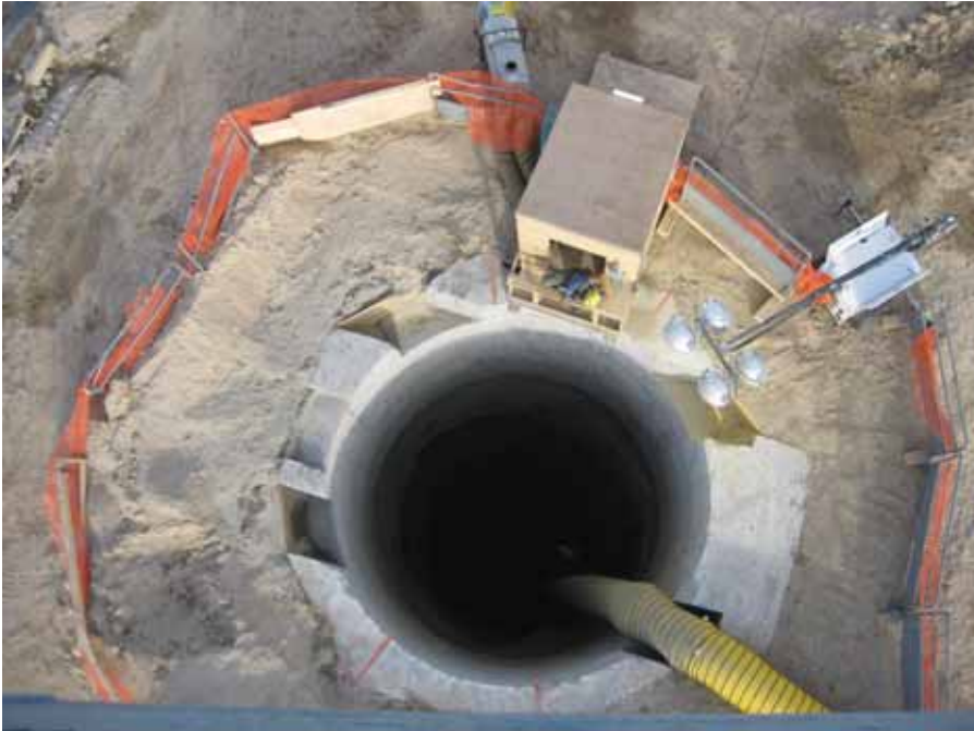
LOOKING DOWN COLLAR – MARCH 2011.
