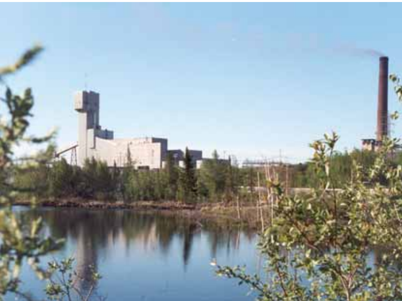
MANITOBA OPERATIONS COMPLETES LATEST PHASE OF UPGRADES TO THEIR THOMPSON MILL WITH SIX NEW OUTOTEC FLOTATION TANK CELLS.
