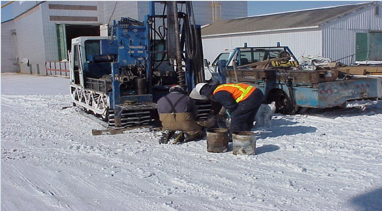
Typical subsurface investigation
