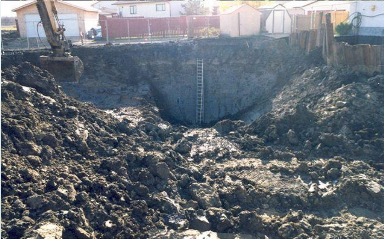
Excavation next to houses
